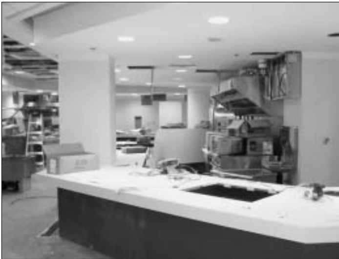
One of the food stations under construction.
